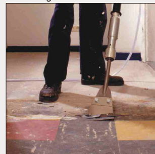
Removal of PVC-tiles
