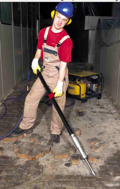
Removing of wood-block paving
