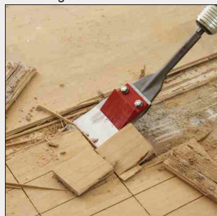
Detaching PU-elastic glued parquet
