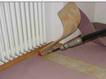
Dismantling carpeted floor coverings
