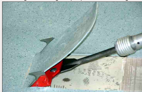
Loosening and cutting soft floor coverings
