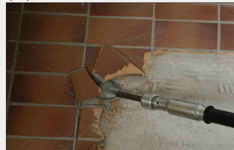
Battering off ceramic floor tiles
