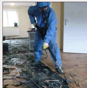
Removing multilayer parquet
