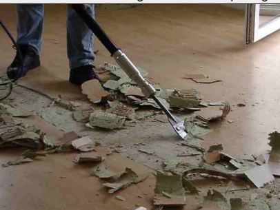
Dismounting elastically glued laminate
