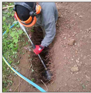
Creating sounding diggings
