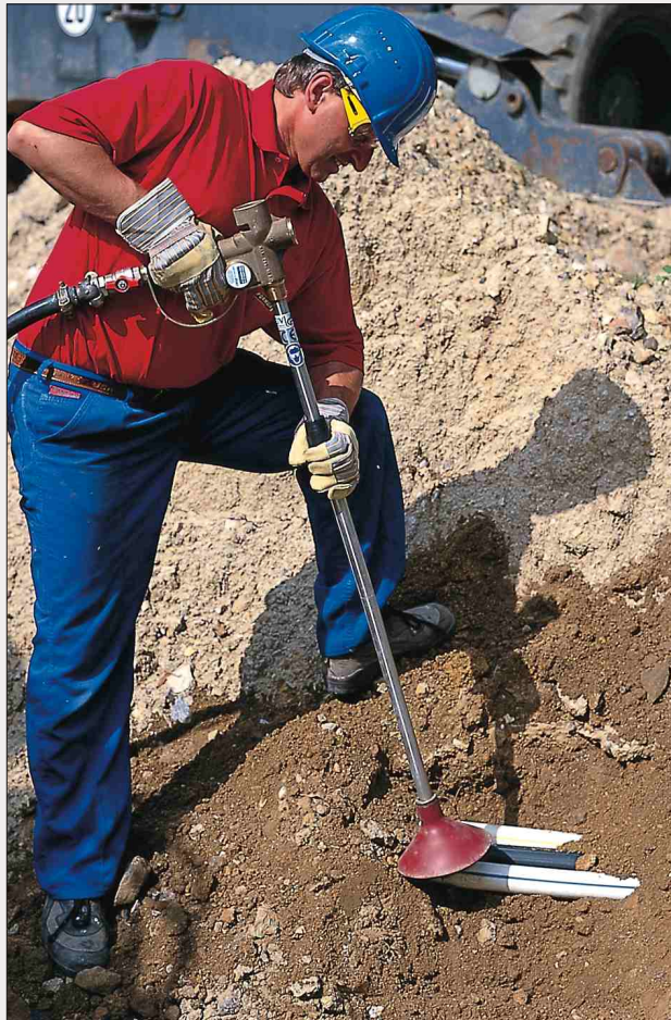
Uncovering of service lines
