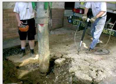
Loosening for suction excavator
