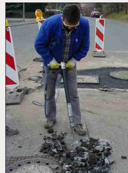
Breaking up asphalt
