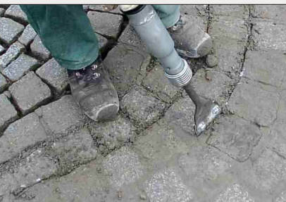
Cutting bounded plaster joints
